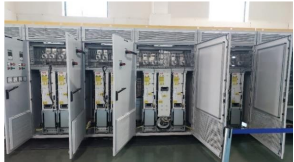
IGBT based ACS880 Drive panels
