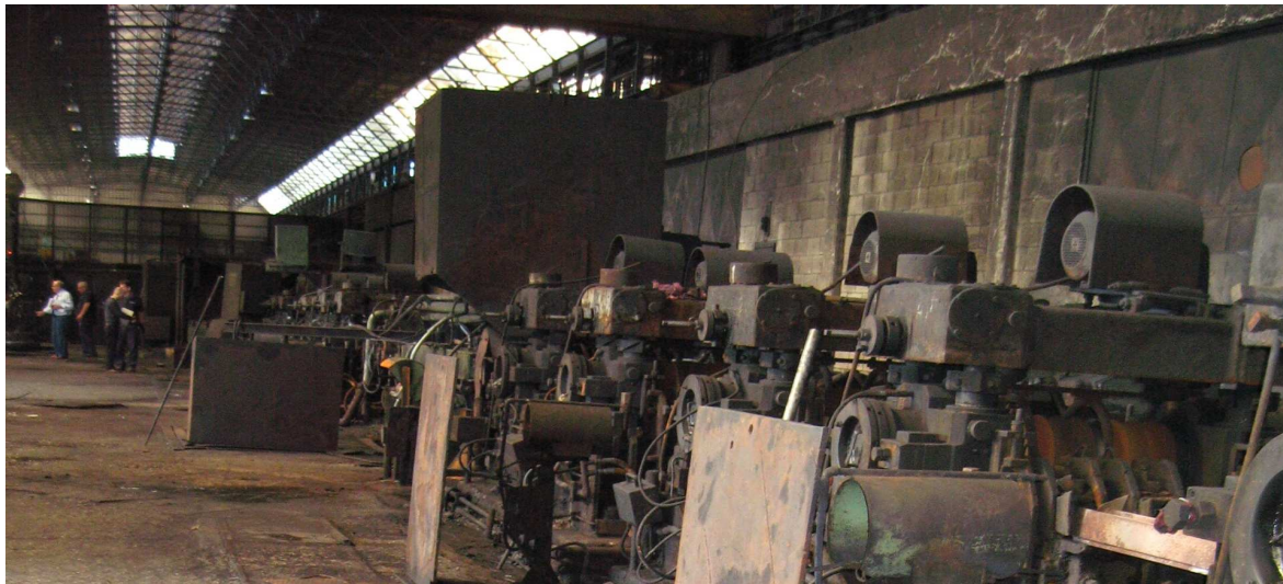
Fig. 2. Collecting of technical data of the plant
